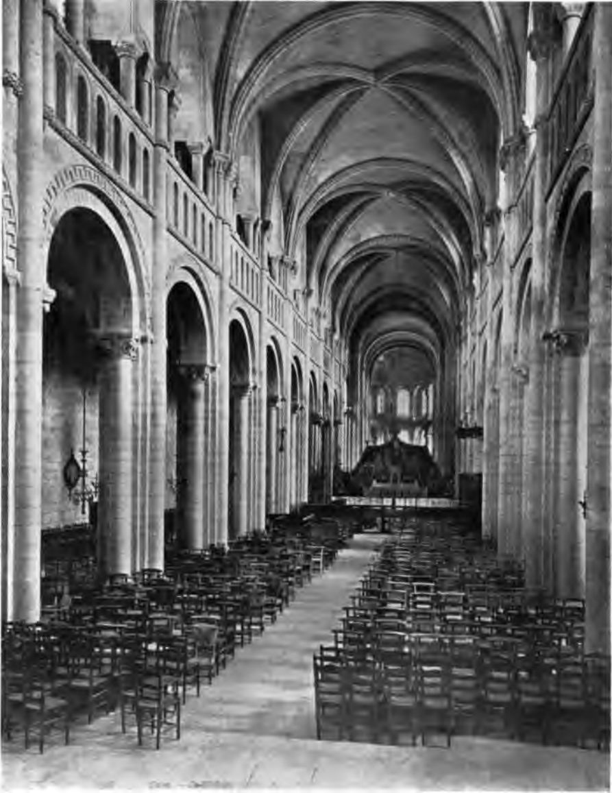
ILL. 128. — Abbaye-aux-Dames of Caen. Interior of Nave
