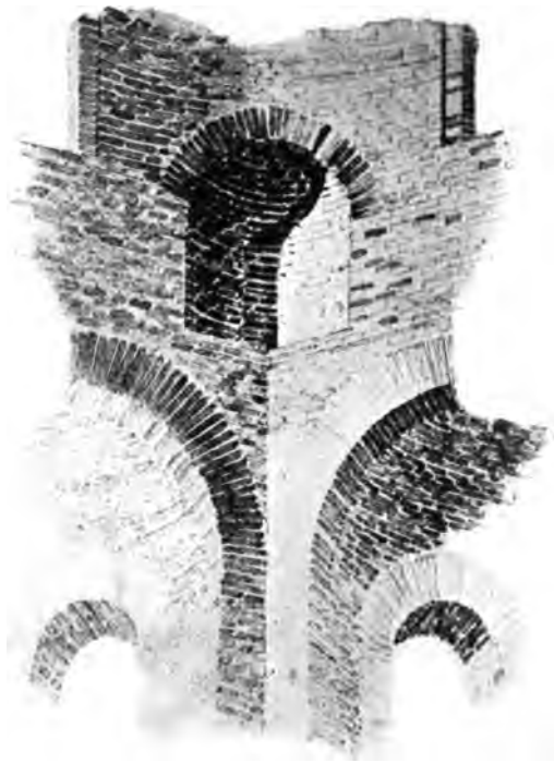
ILL. 76. — Construction of Arched Squinch at S. Vitale, Ravenna. (From Rivoira, by Special Permission)
