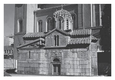
**Figure 12.4** "Little Metropolitan," Athens, ca. 1200. This small cross-in-square church in Athens is unusual in that it was built completely of marble blocks, reused from earlier structures. These blocks include a representation of the ancient goddess Athena, allusions to the cult of Eleusis, and the only surviving depiction of the Panathenaic procession. Many ancient funeral reliefs were also employed, frequently modified to include crosses. Photo: Timothy E. Gregory
