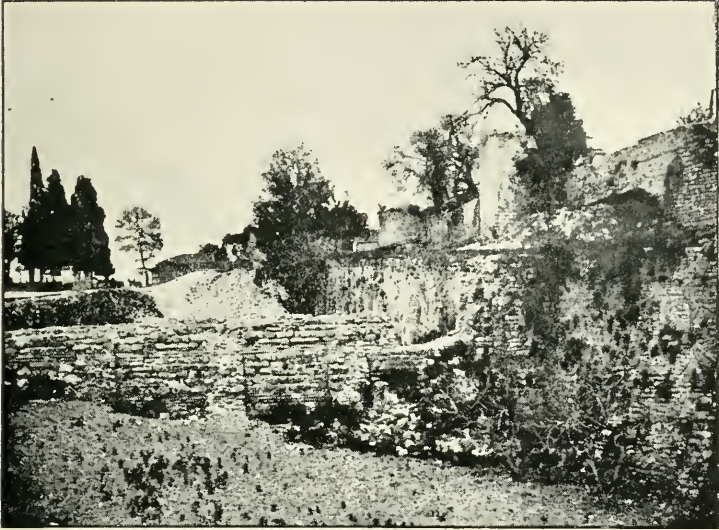
AQUEDUCT ACROSS THE MOAT OF THE THEODOSIAN WALLS.
